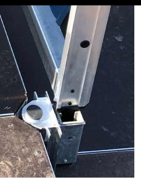
Not all grandstand systems have structural risers. Modular decking systems are also common. With these systems it is not possible to attach seating directly to the system riser.
