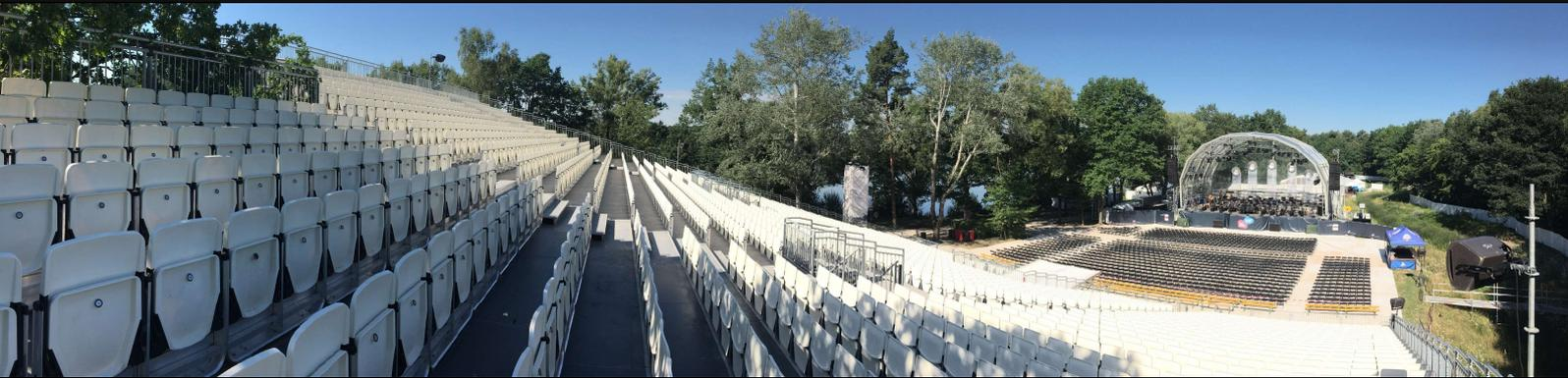
Seating options on these structures ranges from very simple bleachers (benches) which are compact to transport / store and are easy to install but are not very comfortable, though to 'tip up' seating. Conversely 'tip ups' are comfortable but are traditionally bulky requiring special steel cages or 'stillages' in which to transport and store them, they are also awkward to handle and inefficient to install.
