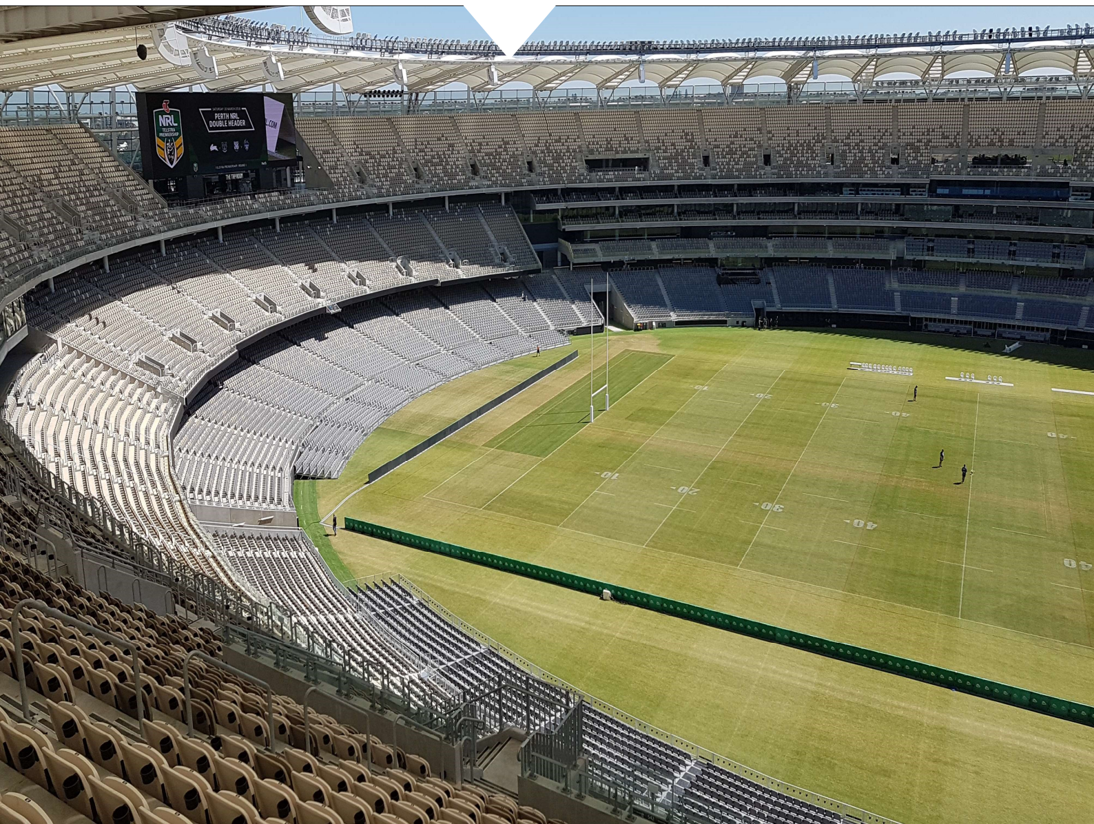
Completed 'drop in' stands for a rectangular event
