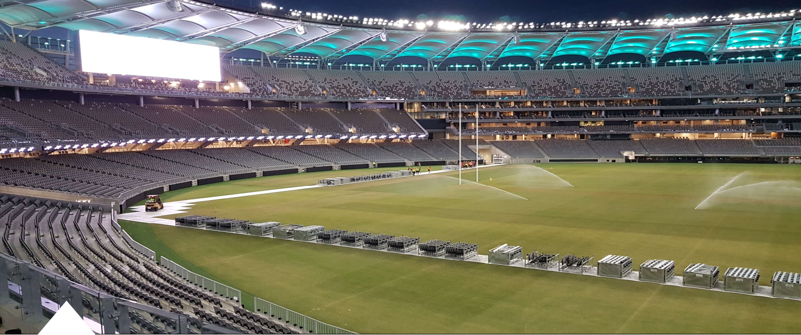
Turf protection in place as multi deck components are laid out for build.
