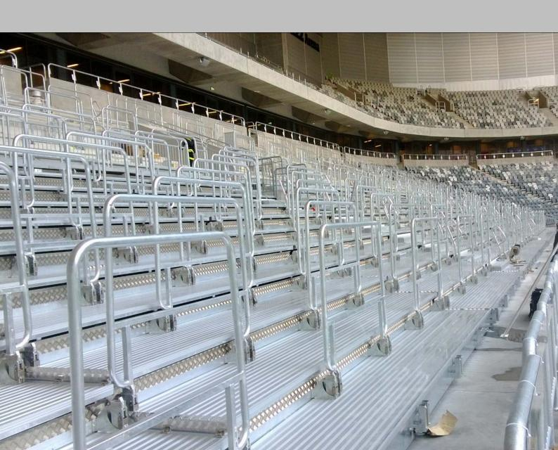
Outdoor - Multi Purpose Arena — Completed in 2013 — will host football — and music events — the telescopic tribune can be set up in seating mode with 1200 solara seat modules — alternatively the seats can be replaced with intermittent crush — rails for standing mode. The Arena has a sliding roof exposing the telescopic to the elements — all materials and finishes were suitable for outdoor conditions.
