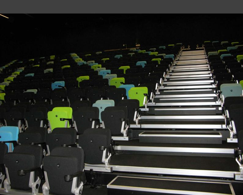
Performing Arts centre – Tivoli is a 800 seat venue – the 18 row telescopic tribune has decra seat modules with full upholstery – the units are power operated and the seats are on semi – automatic fold down mechanisms.
