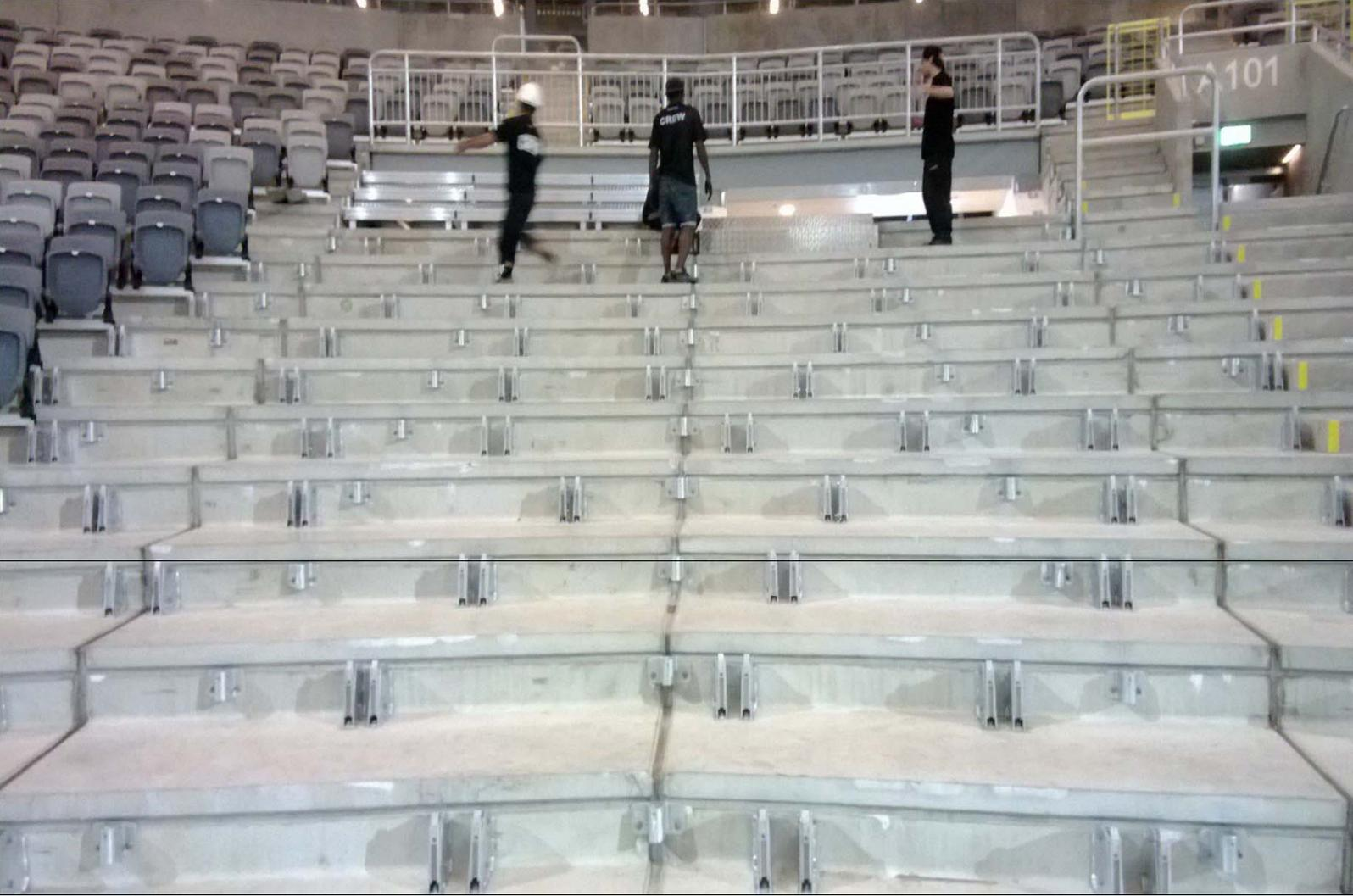
In sport mode these apertures are closed off using a de-mountable structure onto which chairs are mounted - in concert mode they are opened – aluminium step units cover the **fast – latch** mechanisms and lead directly to the playing area.
