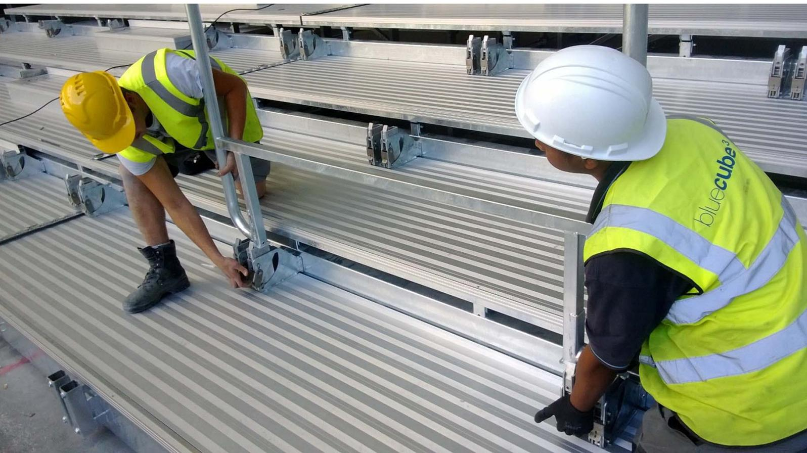
**'P' Rail style post is used in standing mode only to ensure that alternate row end row mechanisms are not a trip hazard.**
