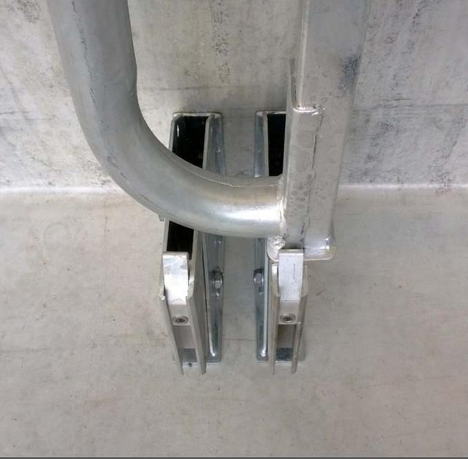
When in standing mode crush rails are intermittent so that the standing crowd has free movement on the terrace – the 'overhanging' design of the crush rail ensures that the adjacent mechanism is made safe and does not cause a trip hazard.
