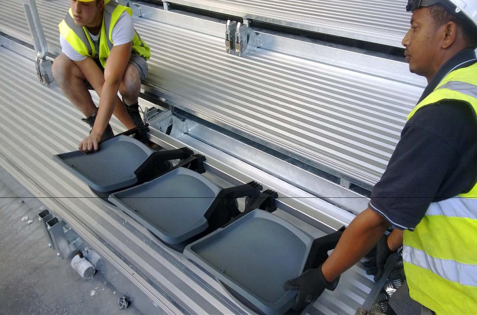
**fast – latch** mechanisms are available with a secondary fold-down function so that they can be used on telescopic units – at the Tele2 Arena the telescopic unit is also used in seating and standing mode – in either seating or crush-rail mode the telescopic can be closed without removing the rails or seats.
