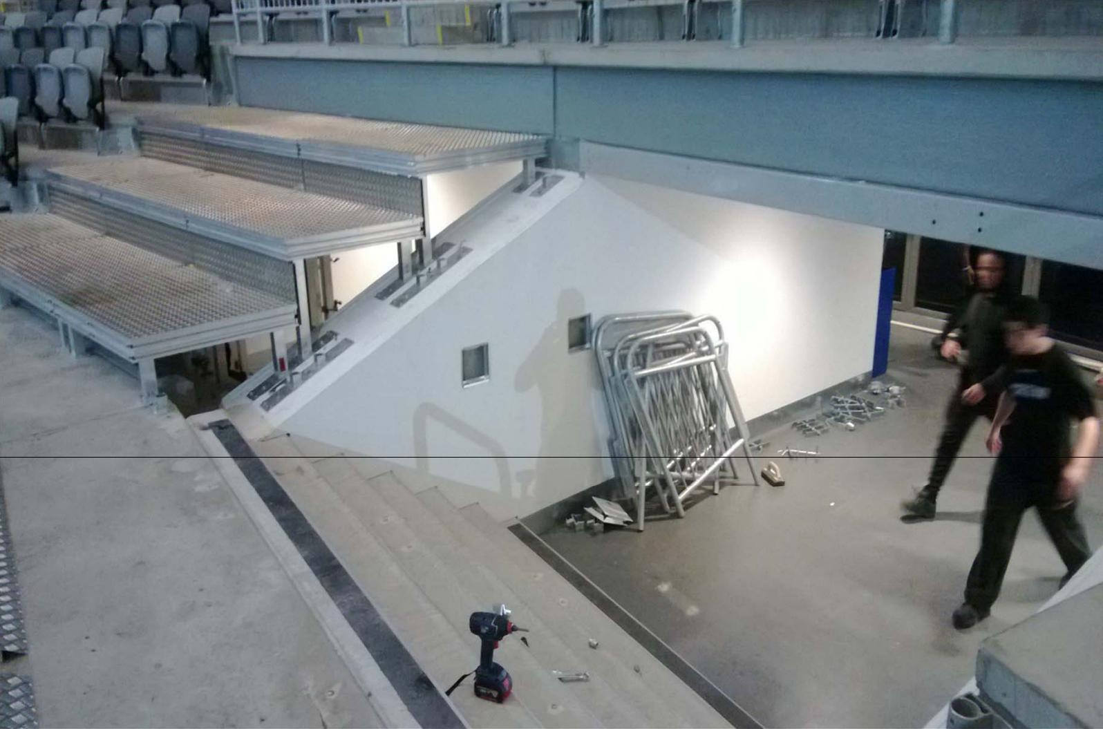
In concert mode the audience will use the playing area to view a performance stage positioned at one end of the arena – this means that larger access routes are required which are built into the lower terrace.
